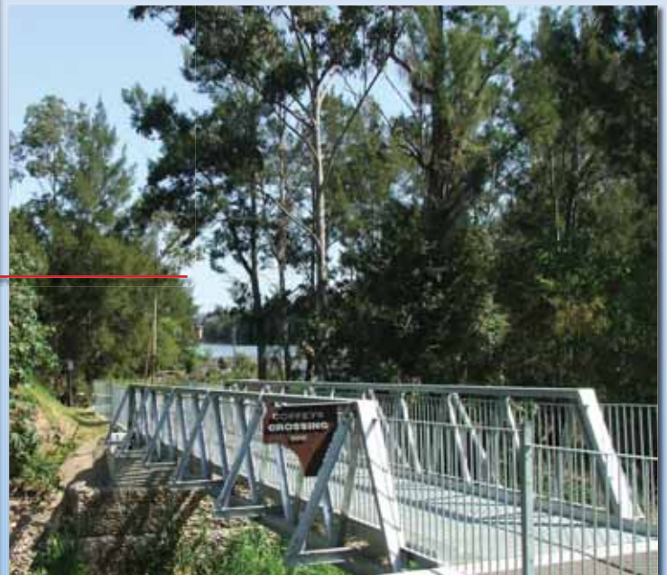
BELOW Providing an all weather crossing of Nepean tributary Boundry Creek was the major engineering work in the new section of the Great River Walk providing previously inaccessible views of Penrith Weir and Victoria Bridge.
